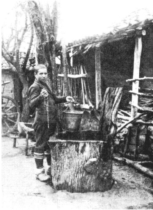
Fig. 4: Reconstruction of a tree-trunk well lining made by stacking two hollowed-out trunk sections (after Hiddink, 2008; Fig. 7.12)
